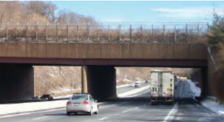
Deer overpass (courtesy of New Jersey Division of Wildlife).
